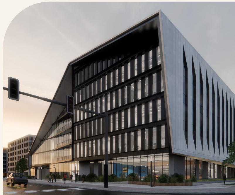
The upcoming 120,000-square-foot Think Dayton facility in Ohio will provide annual STEM education and workforce training to create career pathways for local residents. Source: NBBJ for onMain, Inc.
